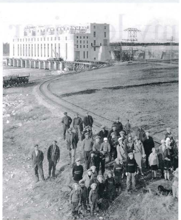
Photo courtesy Manitoba Hydro
